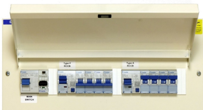
18 th Edition Consumer Unit with Type A and F RCD protection
